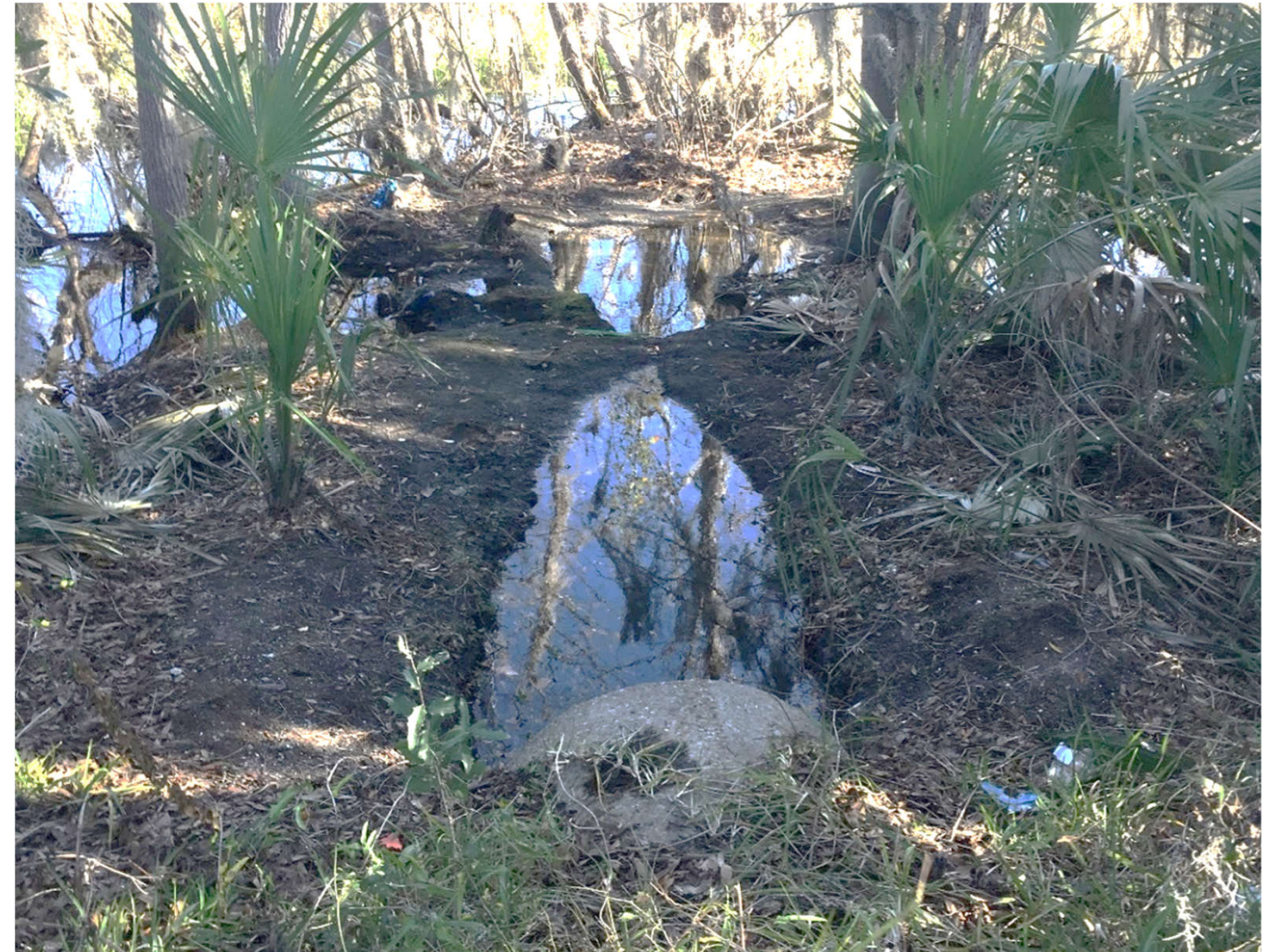
Natural Pond 36" Discharge Pipe (looking into wetland area)
