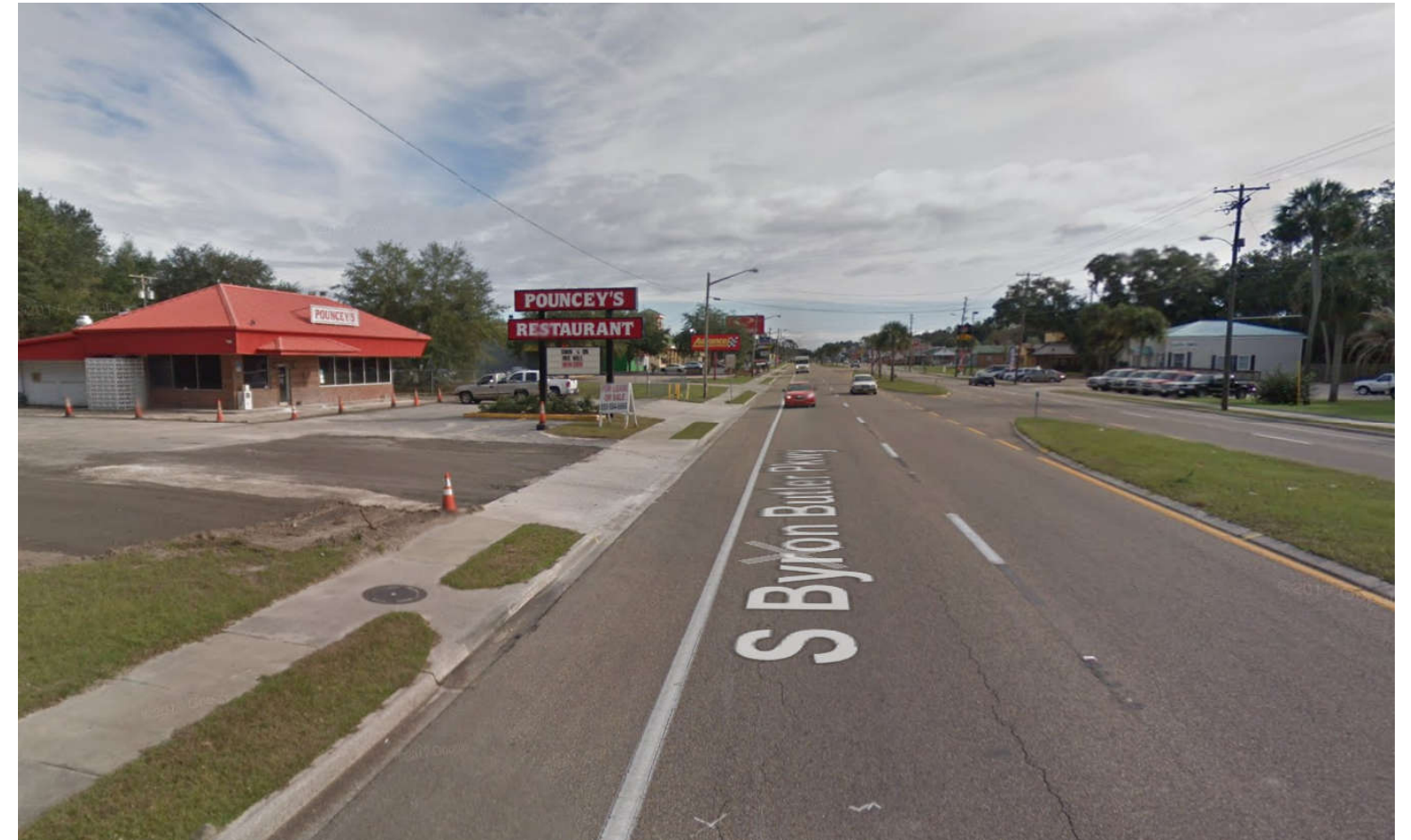
Sag inlet at Pouncey's Restaurant
