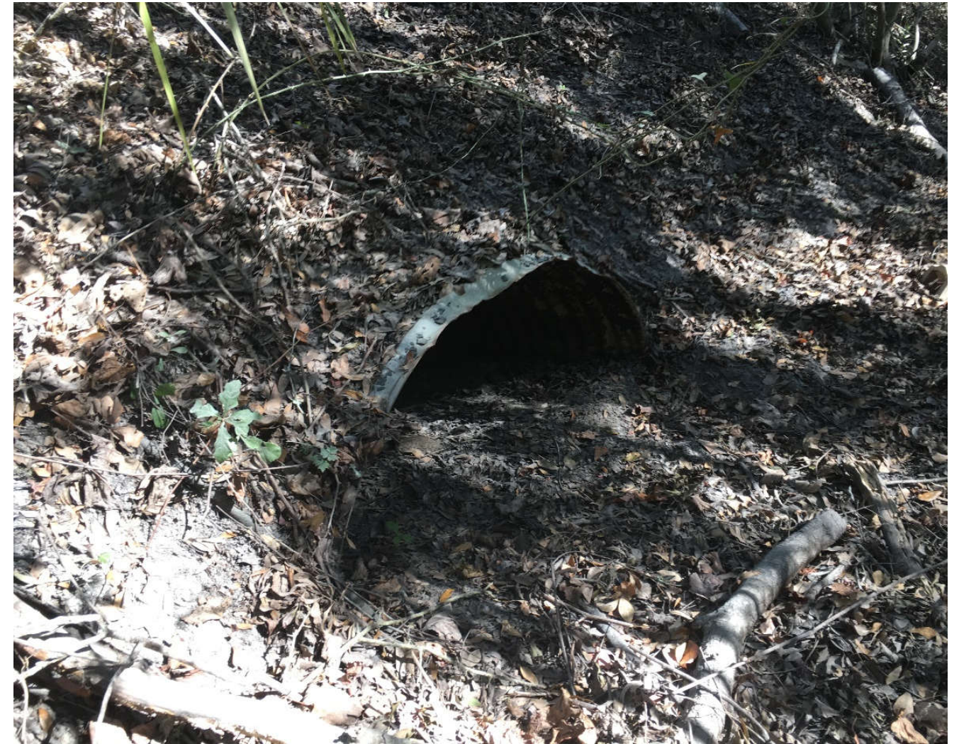
Outfall ditch CMP culverts
