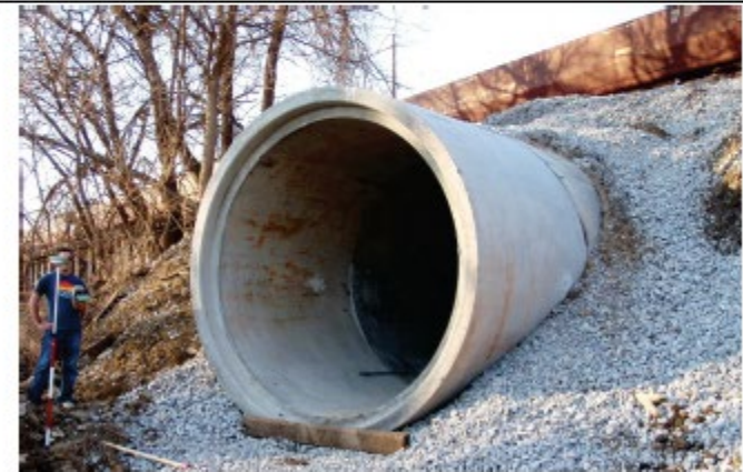
(B) Mitered entrance – The culvert barrel is cut so it is flush with the embankment slope.
