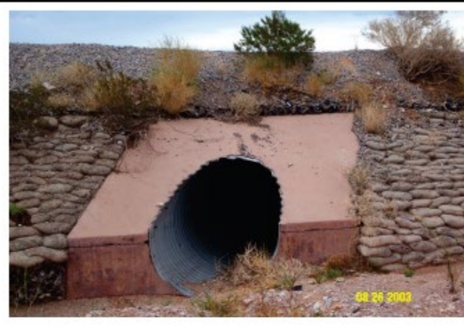
(B) Mitered entrance – The culvert barrel is cut so it is flush with the embankment slope.
