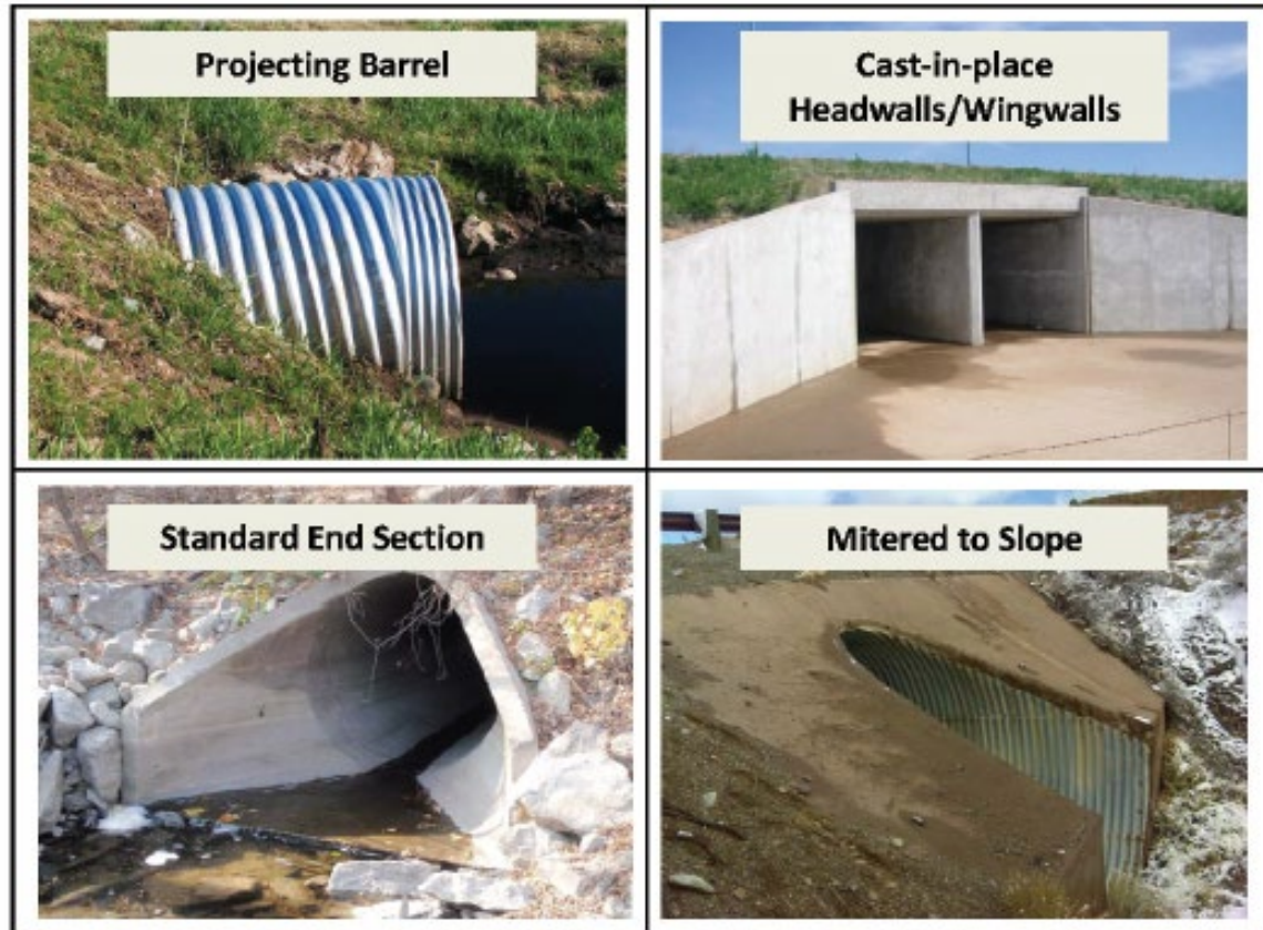
Figure 1.8. Four standard inlet types.
