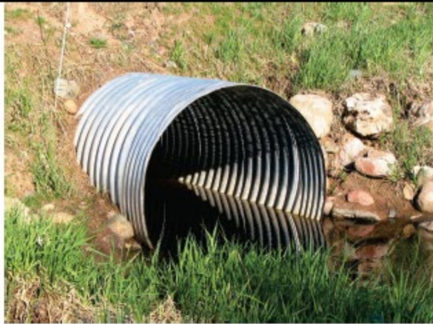
(A) Thin Edge Projecting – The culvert barrel projects out of the embankment.
